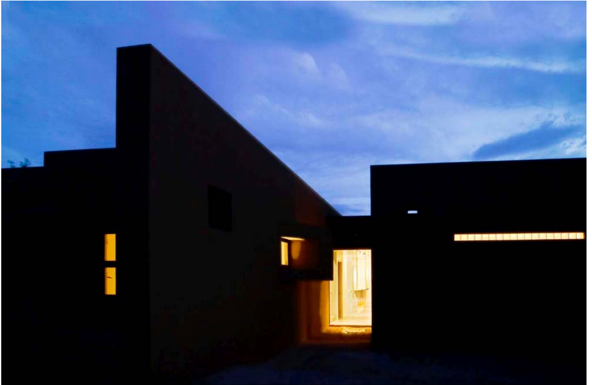
Dynamic wall form emerging on the north side
