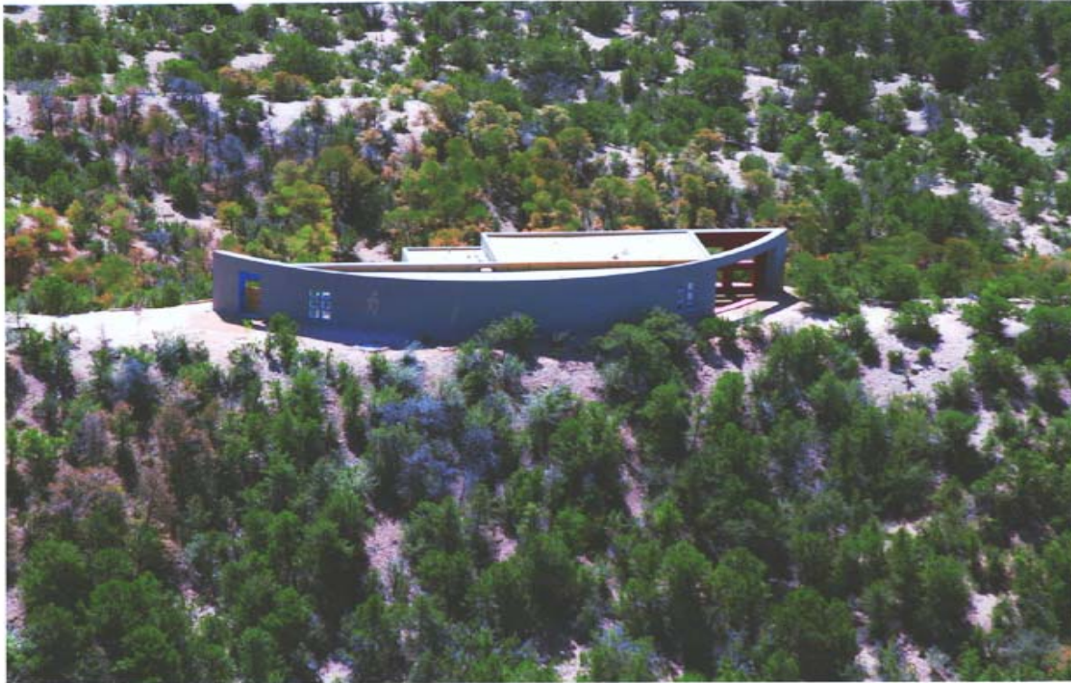
View of the North Curved Wall Library and West Patio
