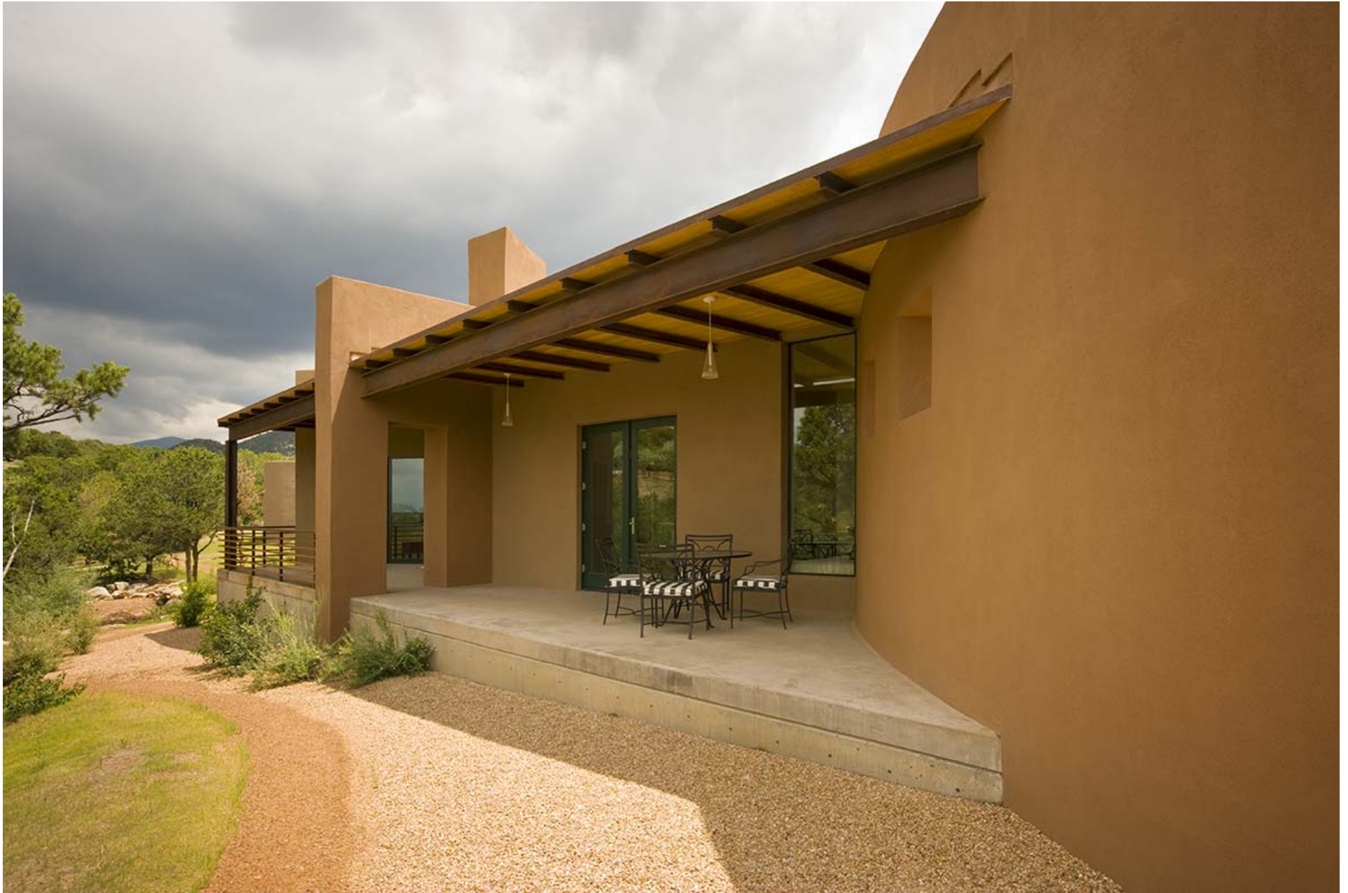
PORTAL INTERSECTING THE CURVES WITH STEEL
