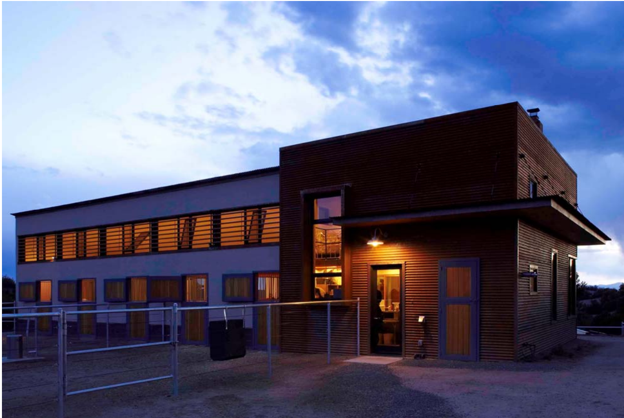
EARLY EVENING PHOTOGRAPH OF SOUTHEAST ELEVATION OF BARN B.
