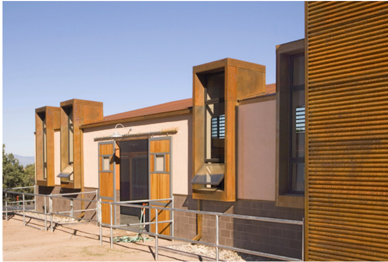
SOUTH ELEVATION OF BARN A. PHOTOGRAPH SHOWS WATER COLLECTORS AT BASE OF WALL. WATER IS HARVESTED FROM ALL THE ROOFS.
