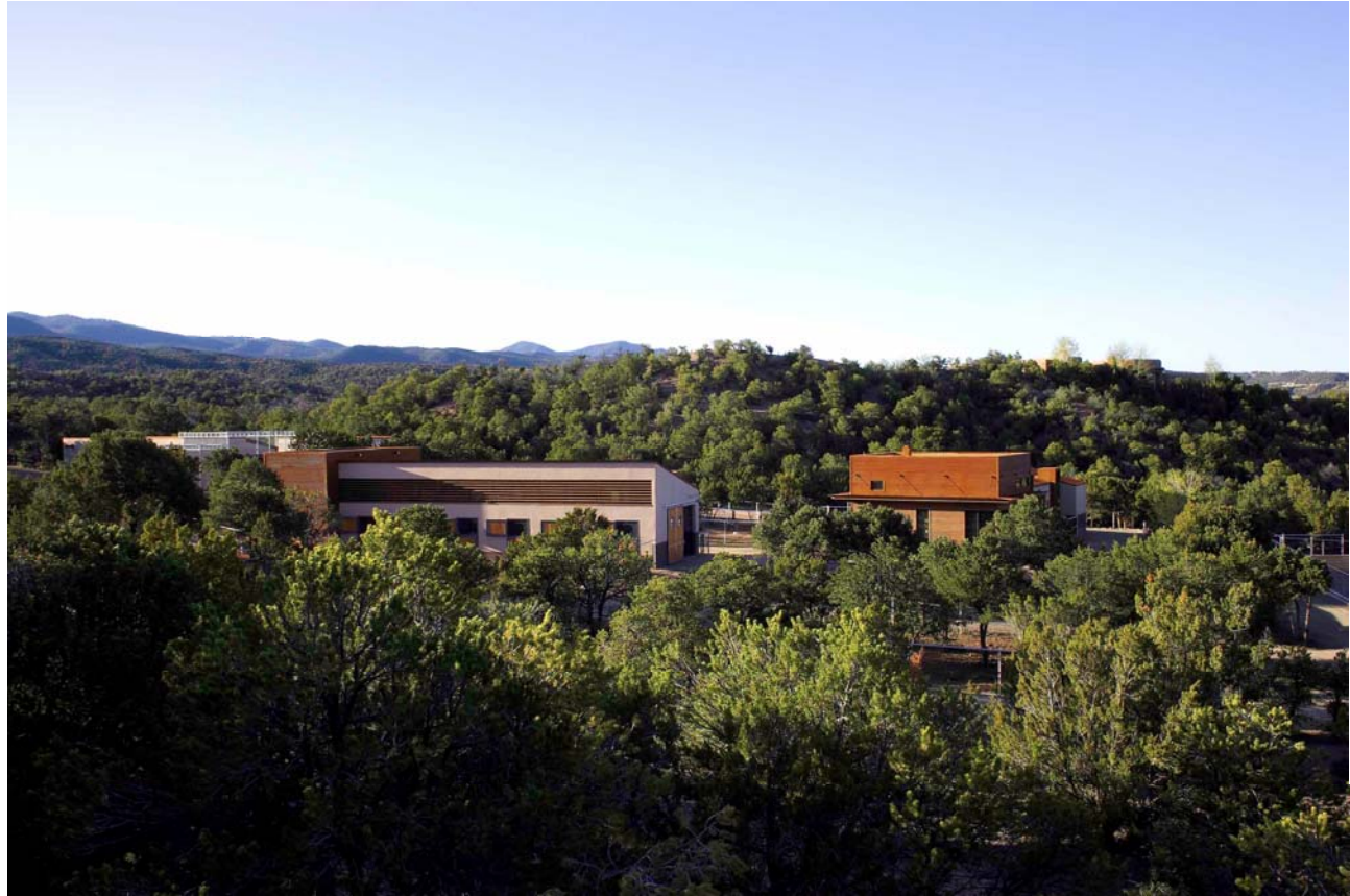
VIEWED FROM THE NORTH NEAR THE ENTRANCE TO THE SITE.
